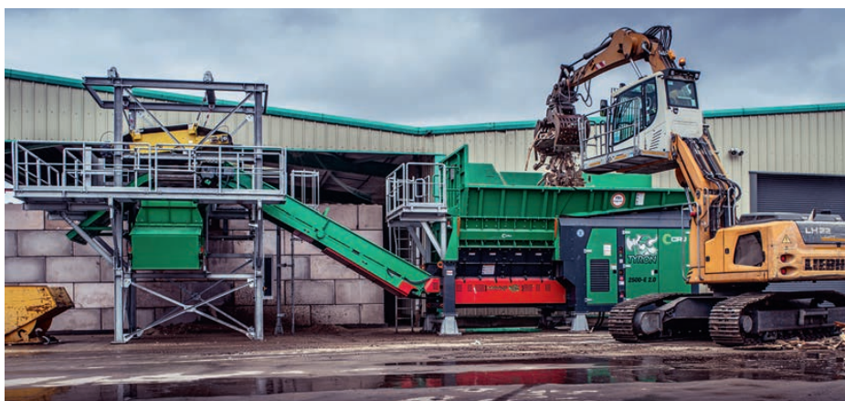
The Leeds2 site, which opened in 2023
